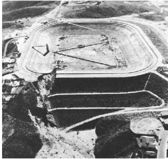
Fig. 1. Piping failure at Baldwin Hills Reservoir, California 1963 (Cedergren, 1967).
